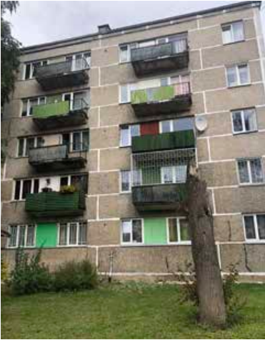
Unrenovated apartment buildings
