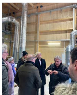
Visit at a highly efficient heating plant
